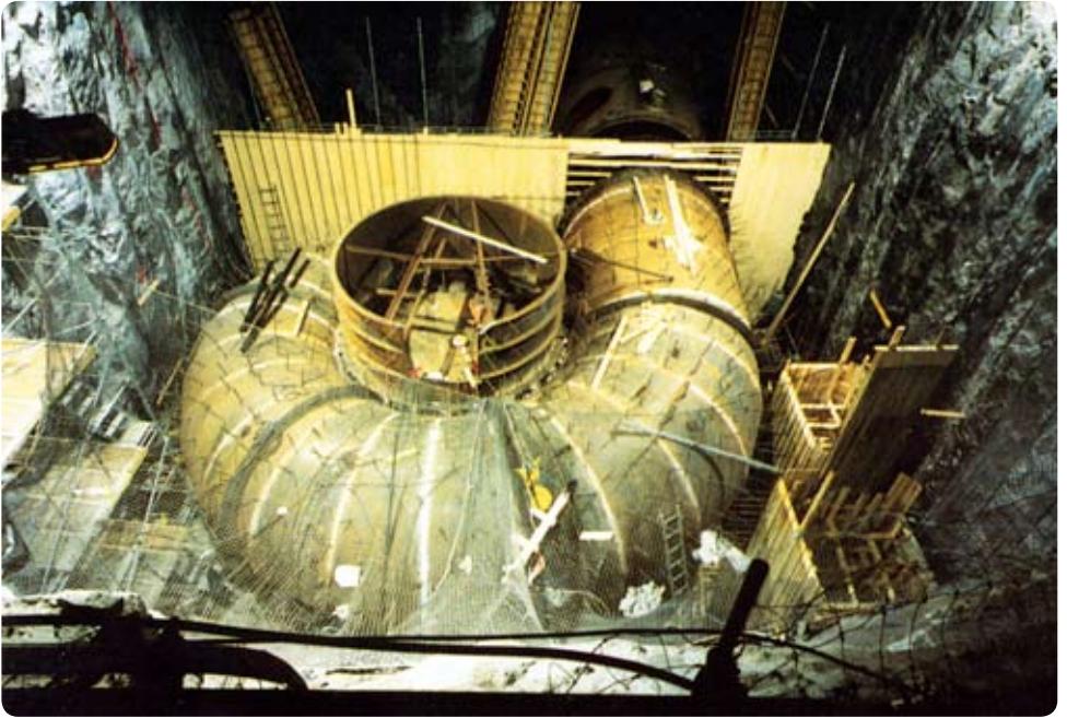
Spiral montage, erection of spiral casing
